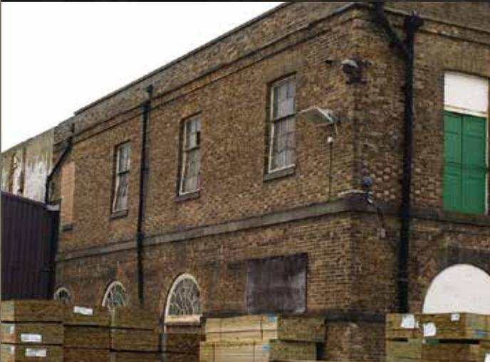
Photos: two external showing the north elevation and the north-east corner (the only window frames still visible – cast iron frames, tilting sashes at 1/F), one internal showing the modular cast iron beams and joists.
